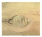
If healthy knots are removed or fall out over time, the hole might need an action according to the maintenance instruction. This should be checked as part of the routine inspection.
