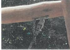
Swing hangers for Robinia wood crossbeams are made of stainless-steel brackets and can move over two axis. The plastic flange bearings are silicone enriched to make the suspension maintenance free.
