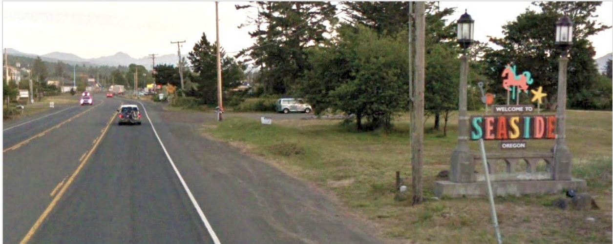
Photograph 6-1. Gateway Treatment Entering Seaside
