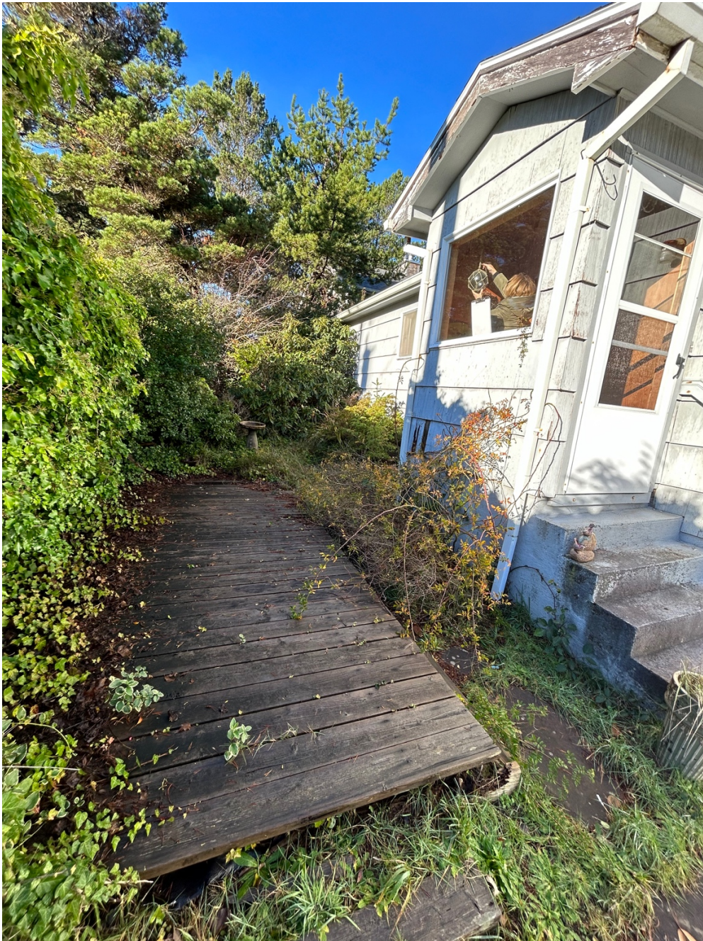
Existing entryway and exterior stair conditions.
